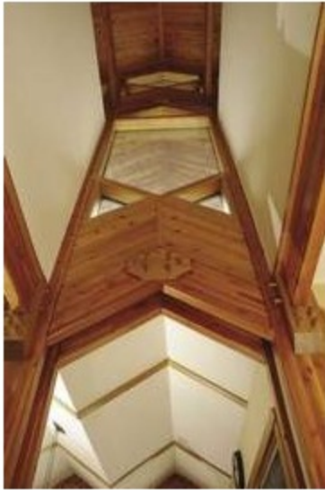
A soaring space adjacent to the kitchen and eating area lets in light and shows off more of the home's frame.
