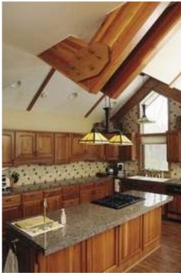
Matt Frideres framed Joe and Lori Redeker's home with enormous laminated beams like the ones in the kitchen.
